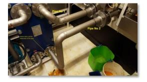
**Problem:** Cooling Pipes supplying the Hydraulic power unit was suffering from internal corrosion resulting in leaks and loss of performance. This vessel operates on a tight schedule, time for repair was limited.
