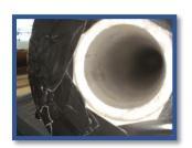
R2 Pipetech's unique lining Epoxy was used to line the HPU Cooling system. The liquid Epoxy was blown through the system to evenly coat the walls of the pipes, forming a smooth barrier between the pipe and water. This barrier coating was then cured before final inspection confirmed that the system was restored to the highest standard of quality.
