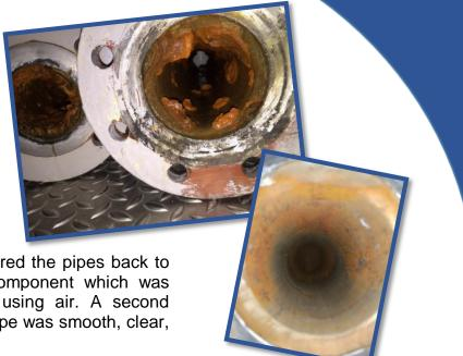
The R2 Pipetech team cleaned and restored the pipes back to their original state using an abrasive component which was shot-blasted through the entire system using air. A second inspection was conducted to ensure the pipe was smooth, clear, and ready for the liner to be installed.
