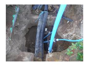
Small diameter pipe (camera entry point)
