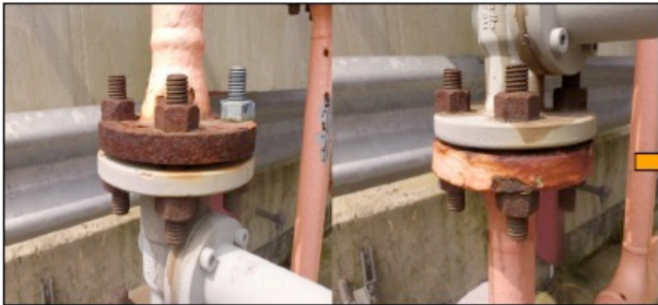
Flanges protected with paint
